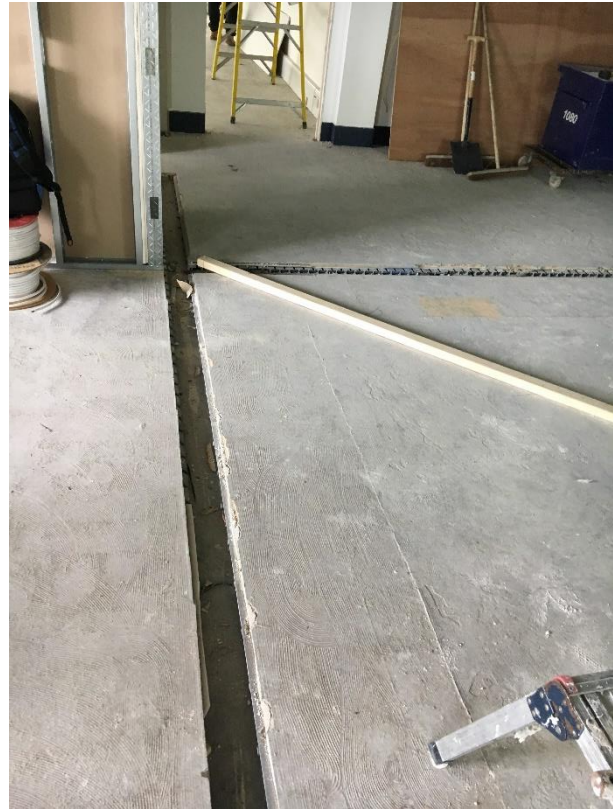
Pre-installed channel can be used to get the cabling from the control box to the first pedestal.
