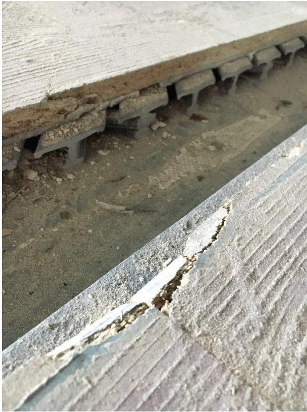
Metal flooring system, not Suitable for under floor cabling or mounting the pedestals.
