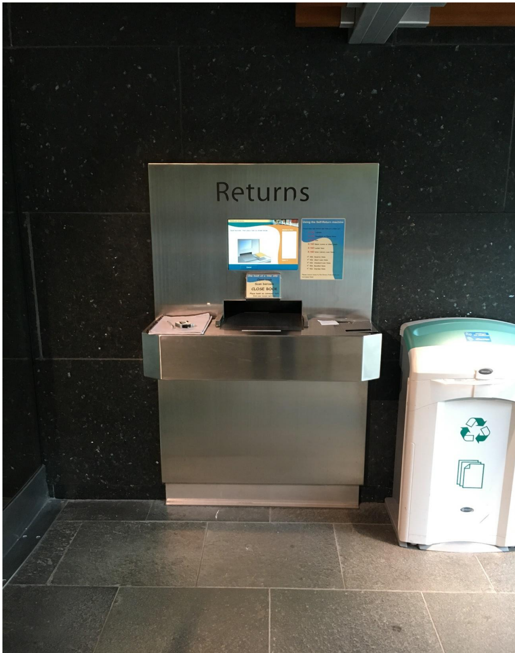
Steel frame that surrounds the infeed unit in the wall.
